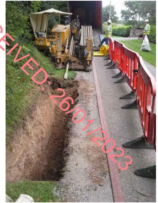
Image 2 : Drilling Rig and Launch Pit
